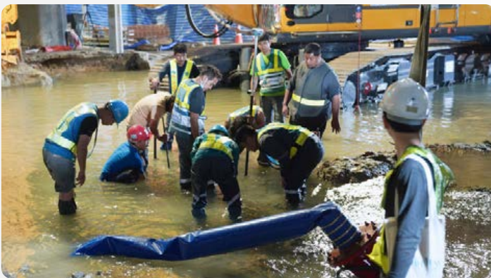
Emergency remediation of damaged distribution main at Ratchaprarop intersection to minimize water disruptions
